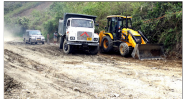
Heavy machinery/vehicles being used for road repair works
